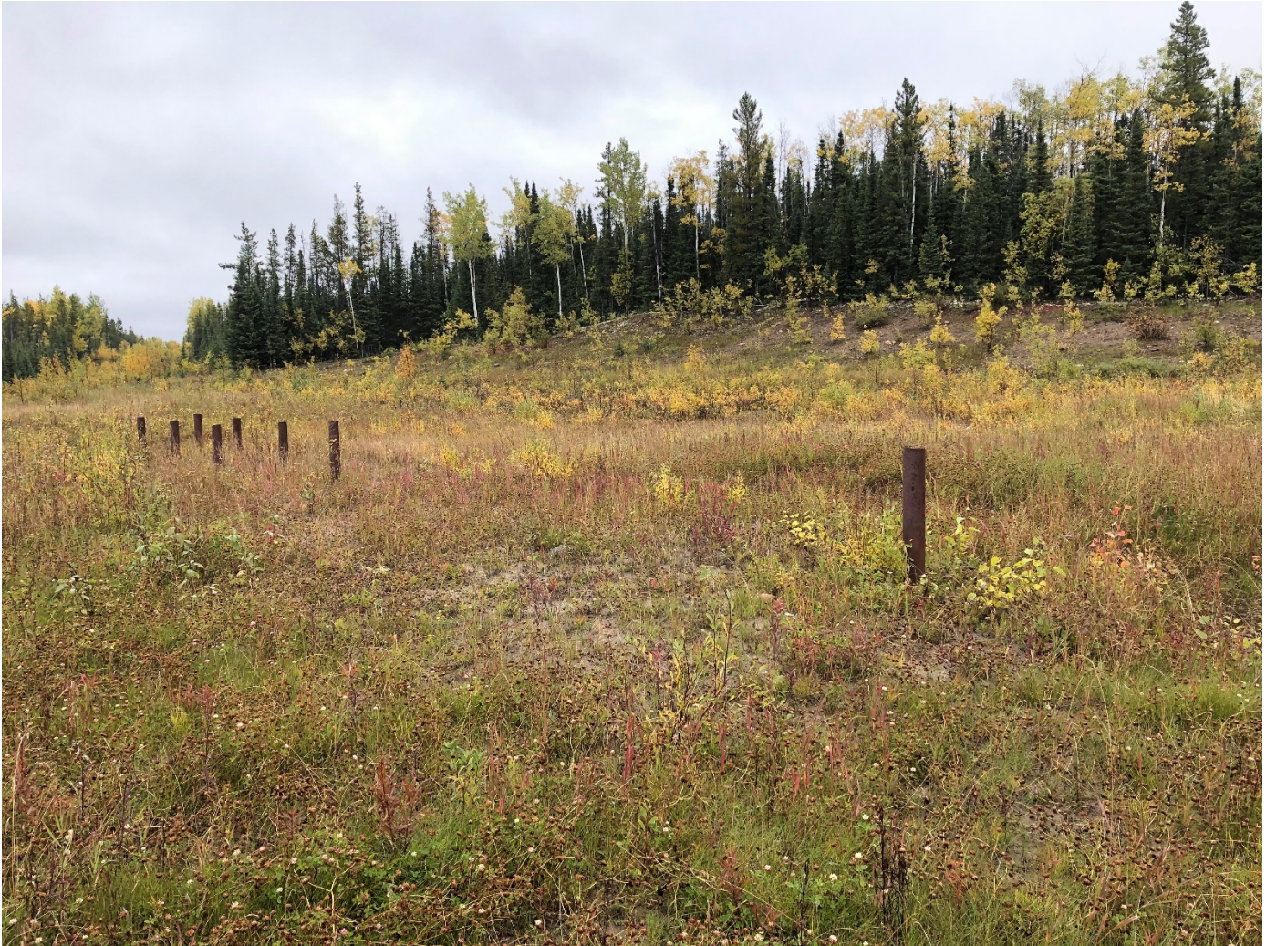
Photo #3: Pilings in place on J-37 well site.
