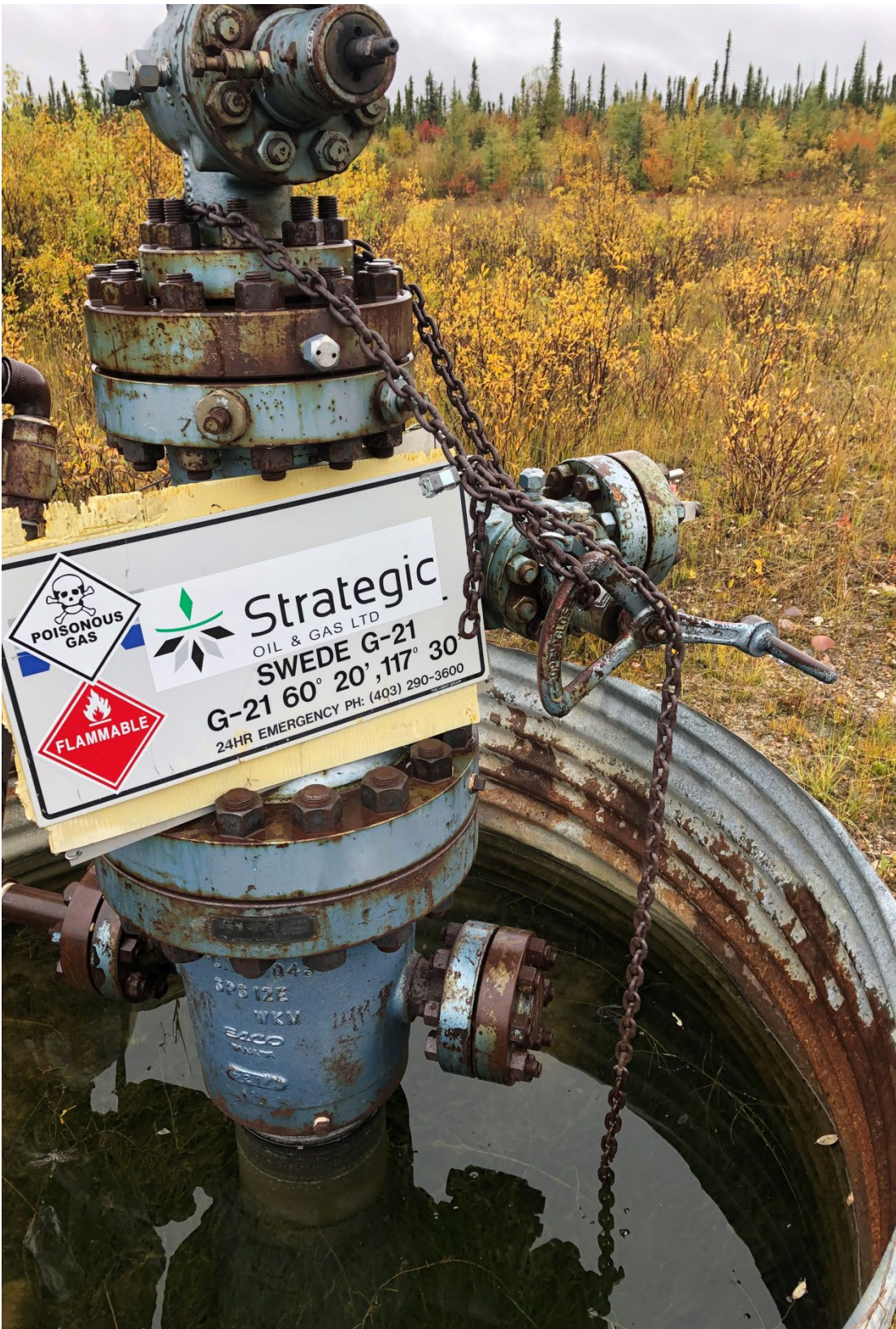
Photo #3: Incorrect 24hr emergency contact number on well sign.
