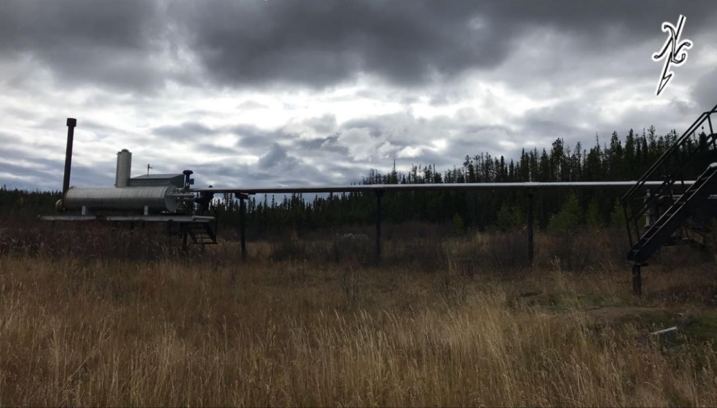
B-38 Well Inspection
