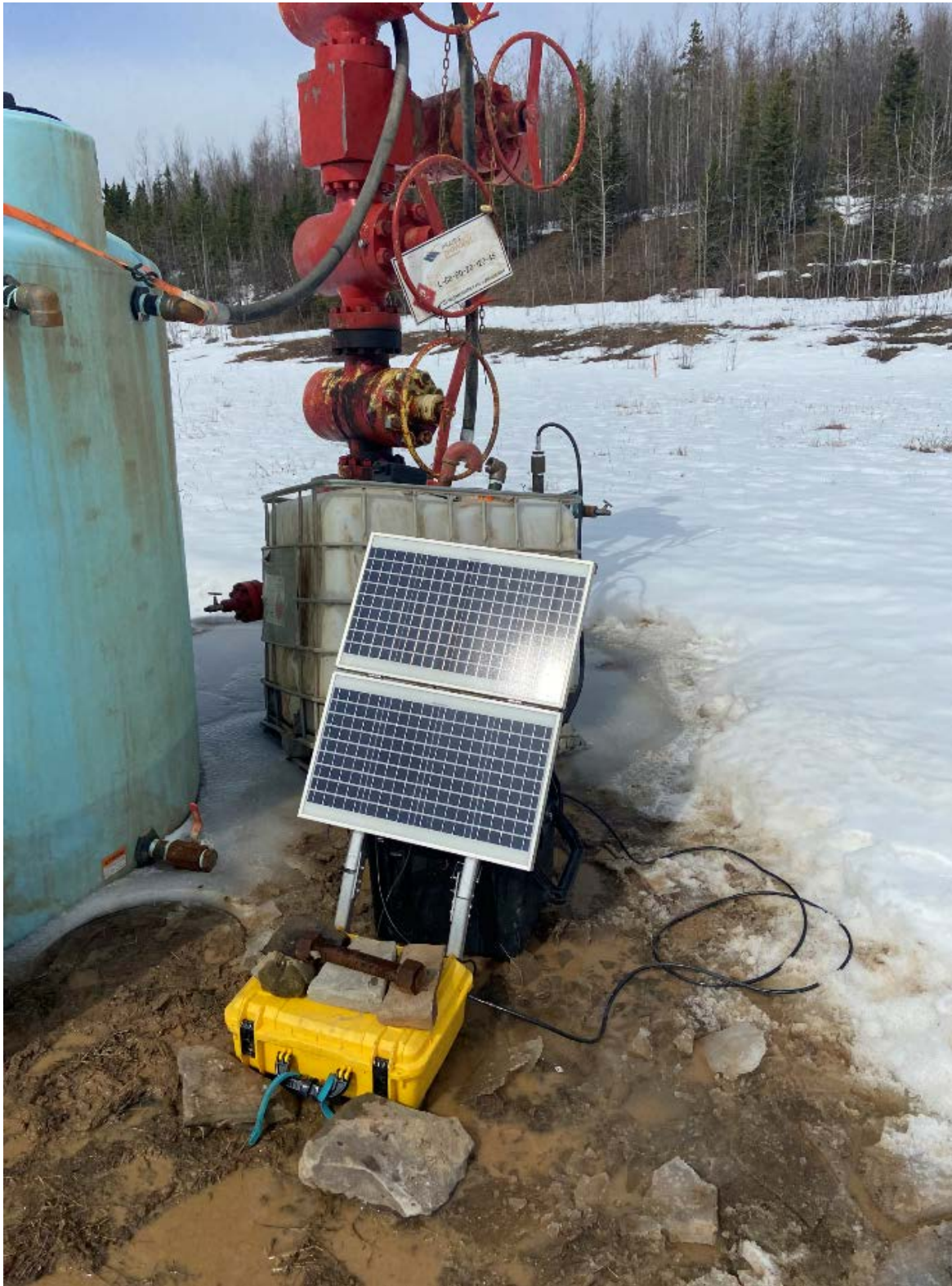
Figure 13 - L-68 SCVF flow meter installation 2021-04-29
